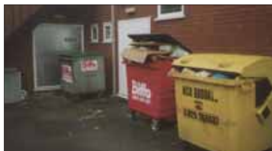
Figure 13: Bins under stairway (courtesy of Cheshire fire service)
