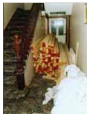
Figure 9: A blocked corridor with incorrect signage
