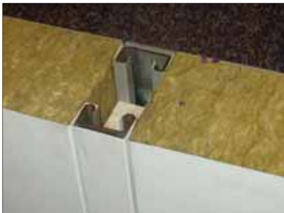
Figure 17: Insulated core panels – internal panel
